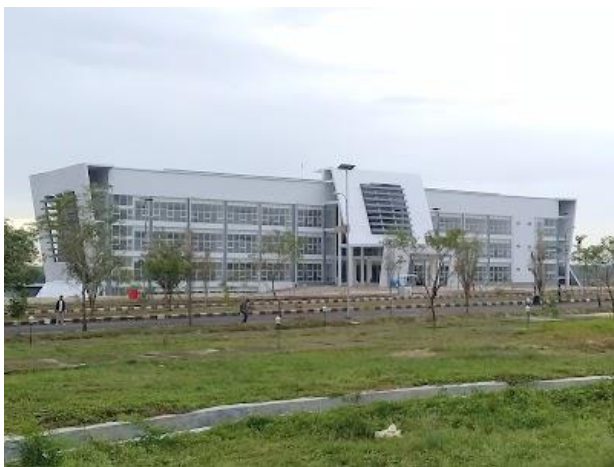
Figure 1. Bandar Lampung building
